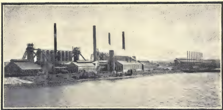
FIG. 59—Blast Furnace at Sydney, C.B.
